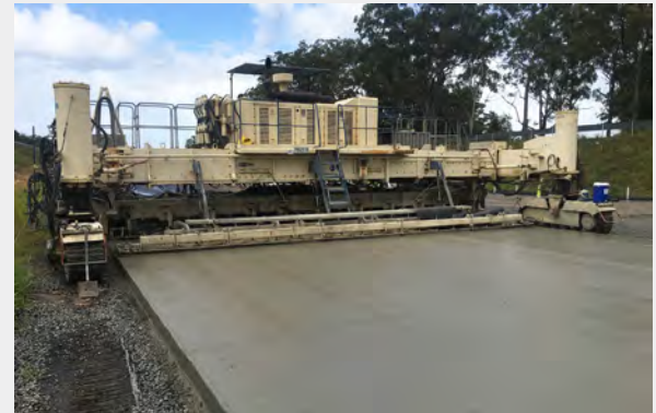
Pavement trial. Photo: © RMS
