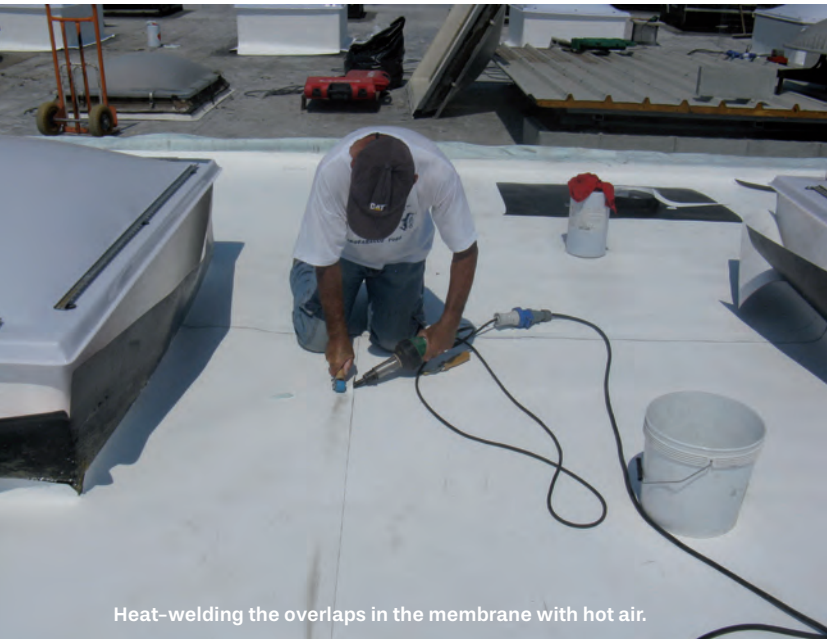
The new skylights covered with Mapeplan T M membranes.
