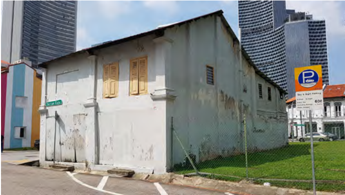
45 Sultan Gate before restoration. Photo: © Singapore Land Authority
